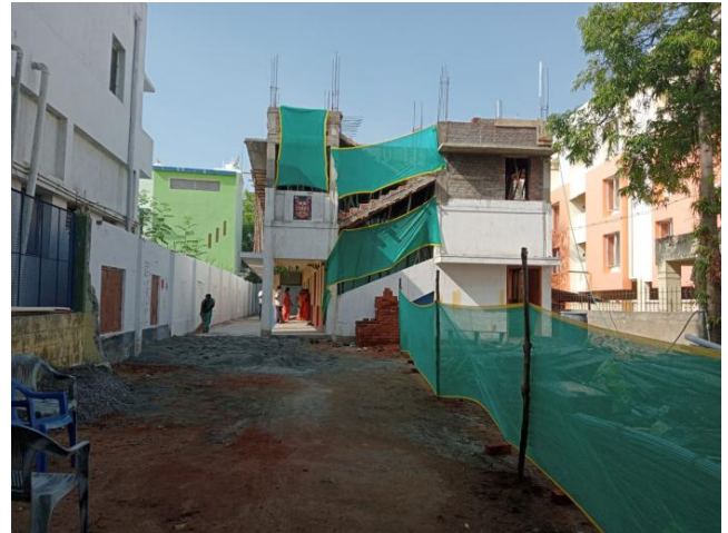
Picture of the new building
